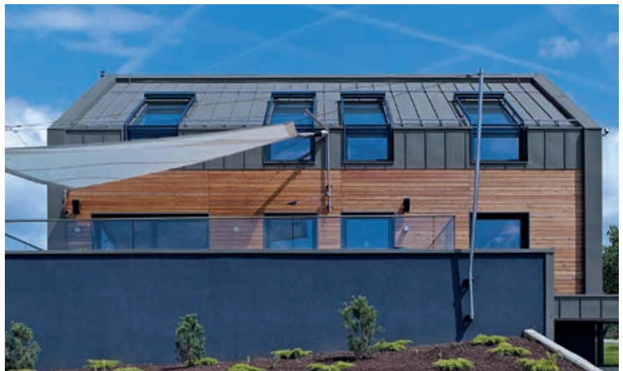
Standing seam covering with roof/facade and gable coping
